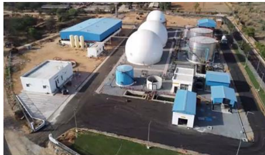
100 TPD Plant at Jaipur Designed By IndianOil
